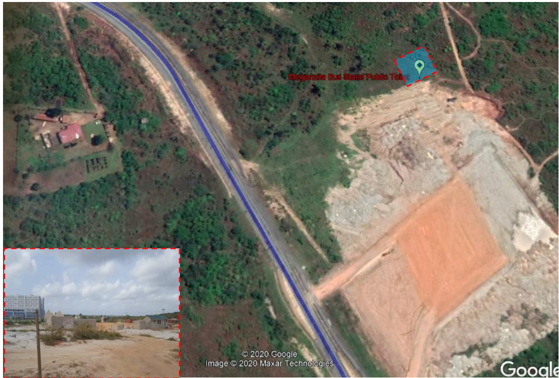
Figure 2: An Extract Google view to show the Location of the project area
